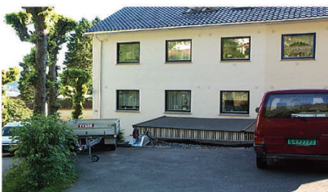
Norwav Exterior Wall
